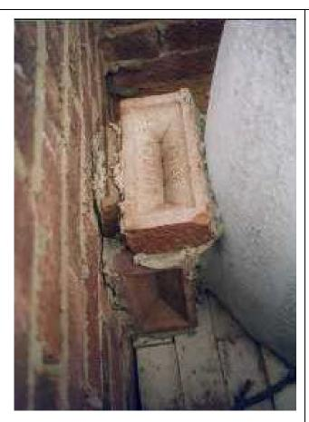
Lift the tandoor liner into the enclosure and check carefully that everything lines up. The air hole must line up with the corresponding hole in the walls and the top of the oven must protrude by 30mm or so above the top course of bricks.
