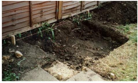
Cut four pieces of wood for the formwork. The pieces should all be 75mm wide. Two should be exactly the length that the slab will be wide, two should be 100mm longer. The short pieces will form two opposite sides of the formwork, as will the long pieces. Cut pegs and screw two pegs to each piece of formwork such that the top of the peg is level with the top of the form.
