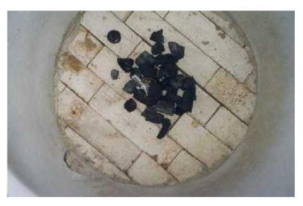
A hot fire might crack the relatively damp liner at this point so be careful to keep the fire small. When the tandoor has cooled check that the liner is still intact and that the fire cement looks secure.
