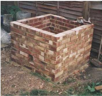
The walls should be exactly a metre square and nine courses high (if your tandoor liner is the same size as mine). The bricklaying is extremely straightforward with the possible exception of the air hole which requires a brick to be cut using the brick bolster (or trowel if you're man enough – you'd better buy extra bricks if you're going to try!).
