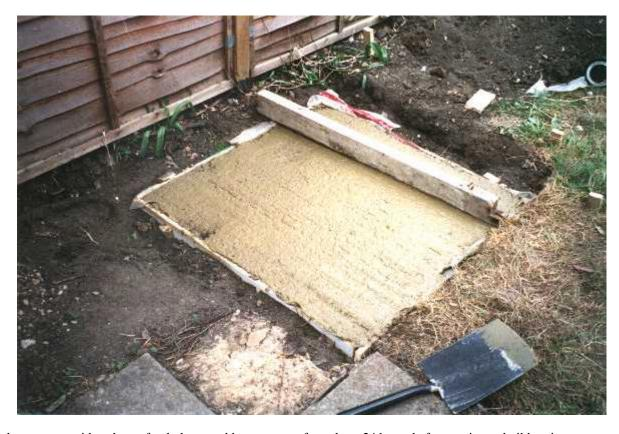
Cover the concrete with a sheet of polythene and leave to cure for at least 24 hours before staring to build on it.
